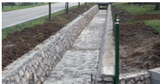
Photo 12 - Improvement of the banks and base of the irrigation channel
