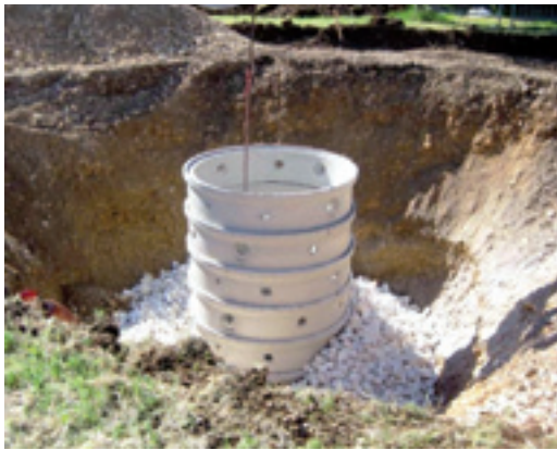
Photo 4 and Figure 4 - Photo and diagram of infiltration well
