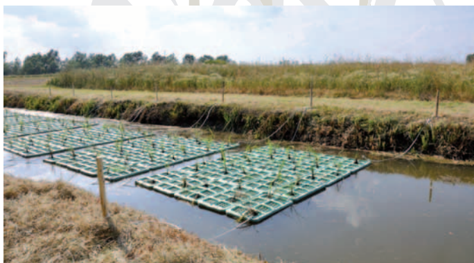
Figure 3 – Anchoring the floating platforms to the bank of the drainage channel with cables.
