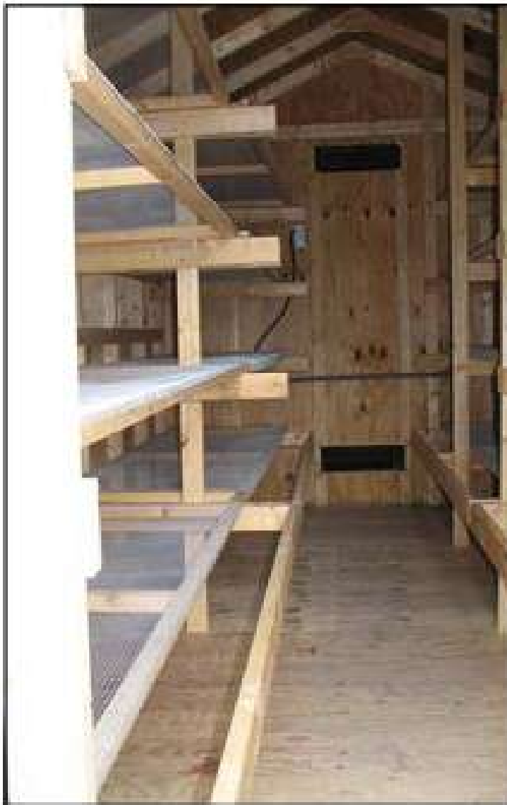
Figure 8: Unfinished frames with shelves installed.
